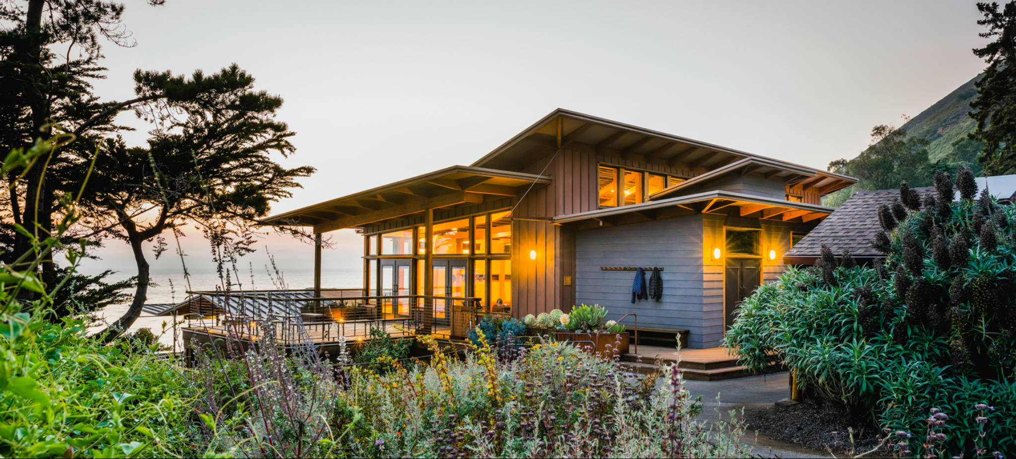
Esalen Lodge Renovation and Expansion
