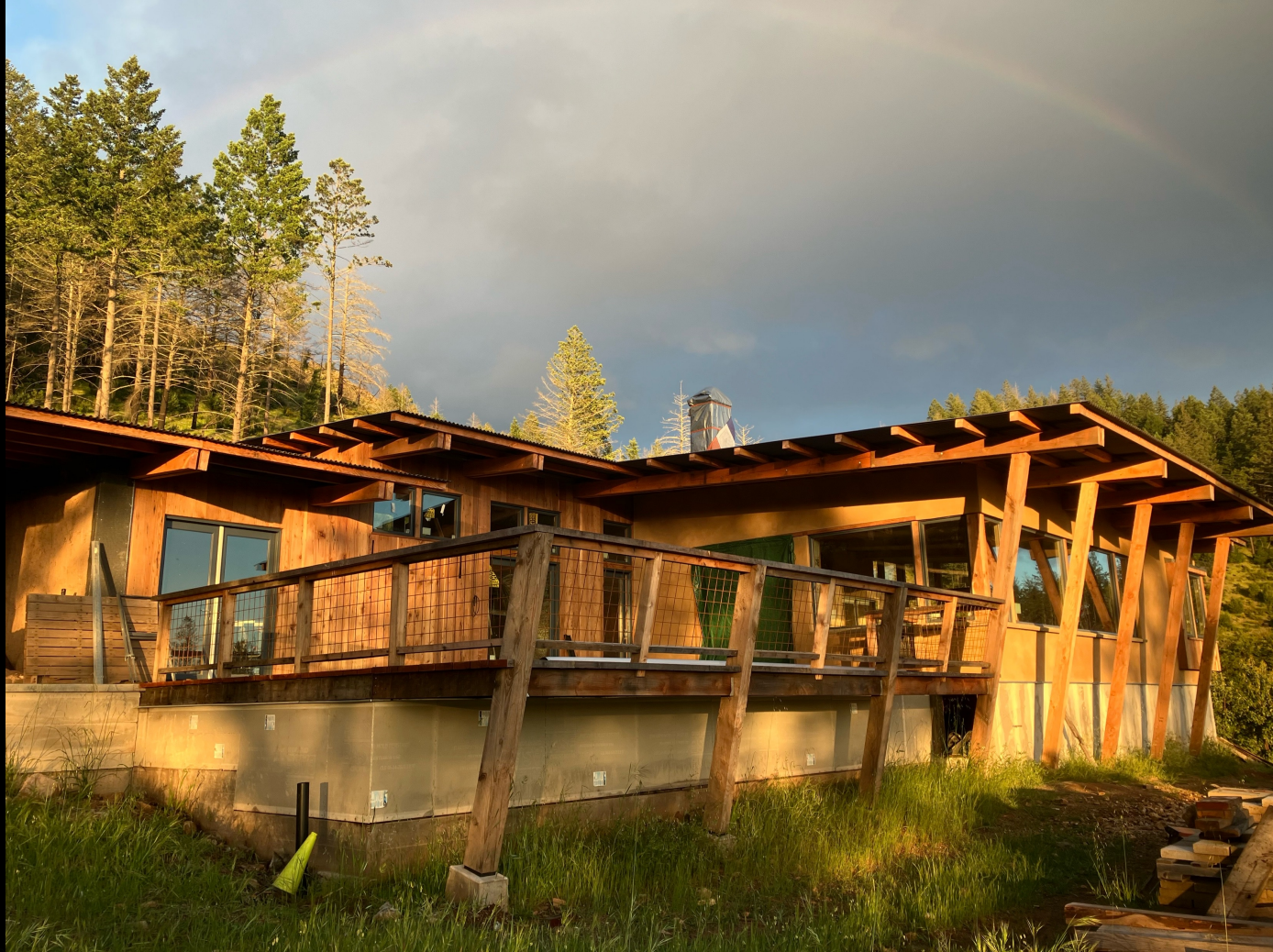
N22 Pythian Road Fire Rebuild, Santa Rosa, CA – Arkin Tilt Architects
