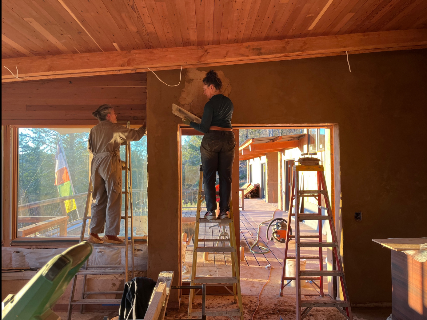
N22 Pythian Road Fire Rebuild, Santa Rosa, CA – Massey Burke / Clay Plaster
