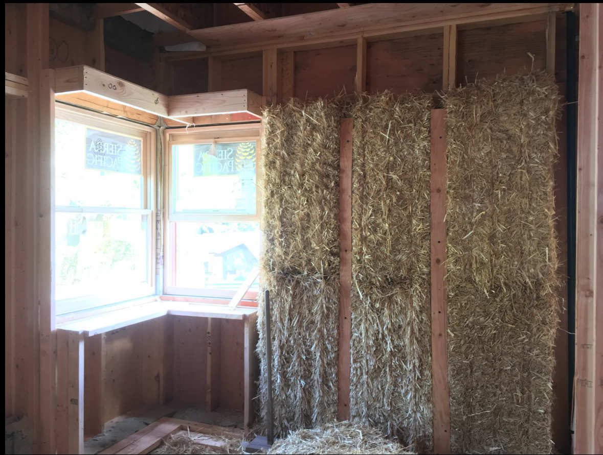
BOEBS – Bales On End Between Studs
